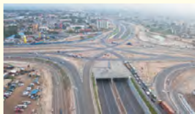
Tema intersection (part of the Ghana International Corridor Improvement Project) (Ghana)
