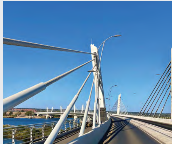
Figure 30: Photo: Kazungula Bridge (AUDA-NEPAD)
